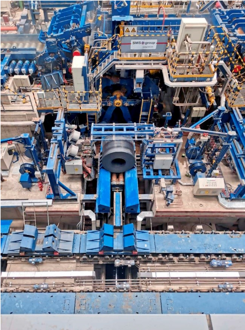
One of three down coilers at the new high-performance hot strip mill of HBIS Laoting.
