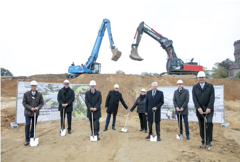
From left to right: Torsten Heising (CFO, SMS group GmbH), Holger P. Hartmann (architect and general planner), Hans Wilhelm Reiners (Mayor of the City of Mönchengladbach), Peter Peskes and Elke Paul (works council chairpersons), Heinrich Weiss (Chairman of the Shareholders' Committee of SMS Holding GmbH), Marco Kubiak (project manager), Burkhard Dahmen (CEO, SMS group GmbH).
