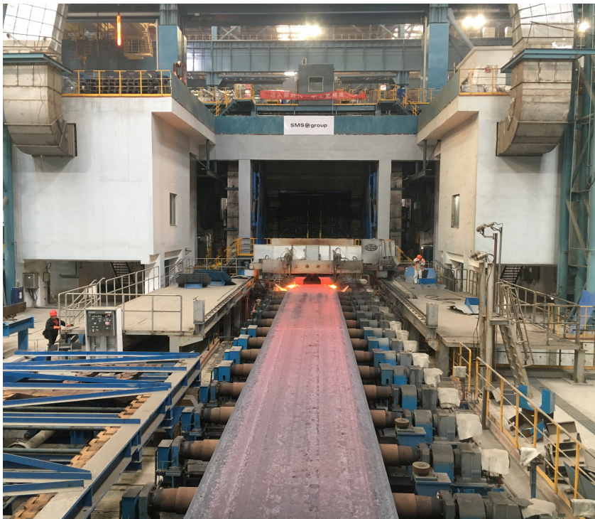
The first slab produced on the new continuous caster.
