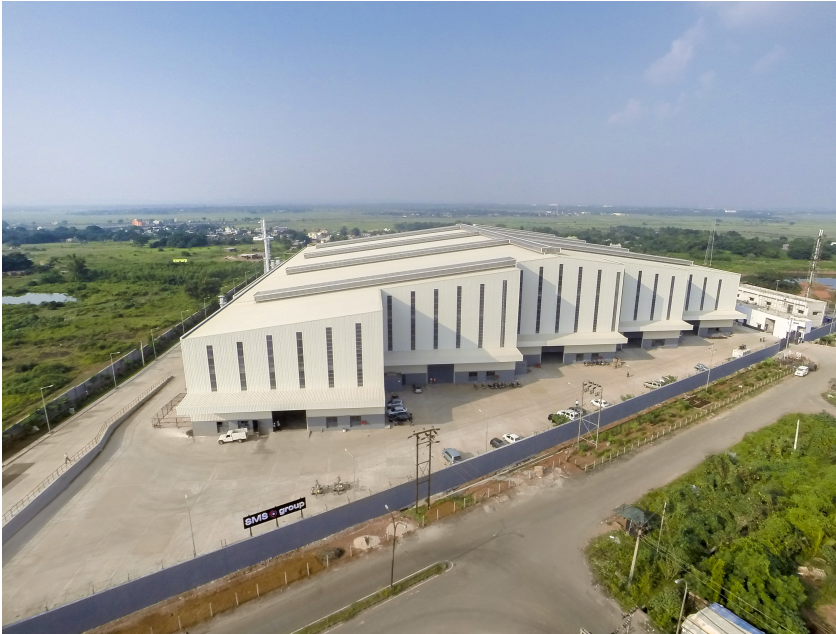
Exterior view of the workshop at Bhubaneswar.
